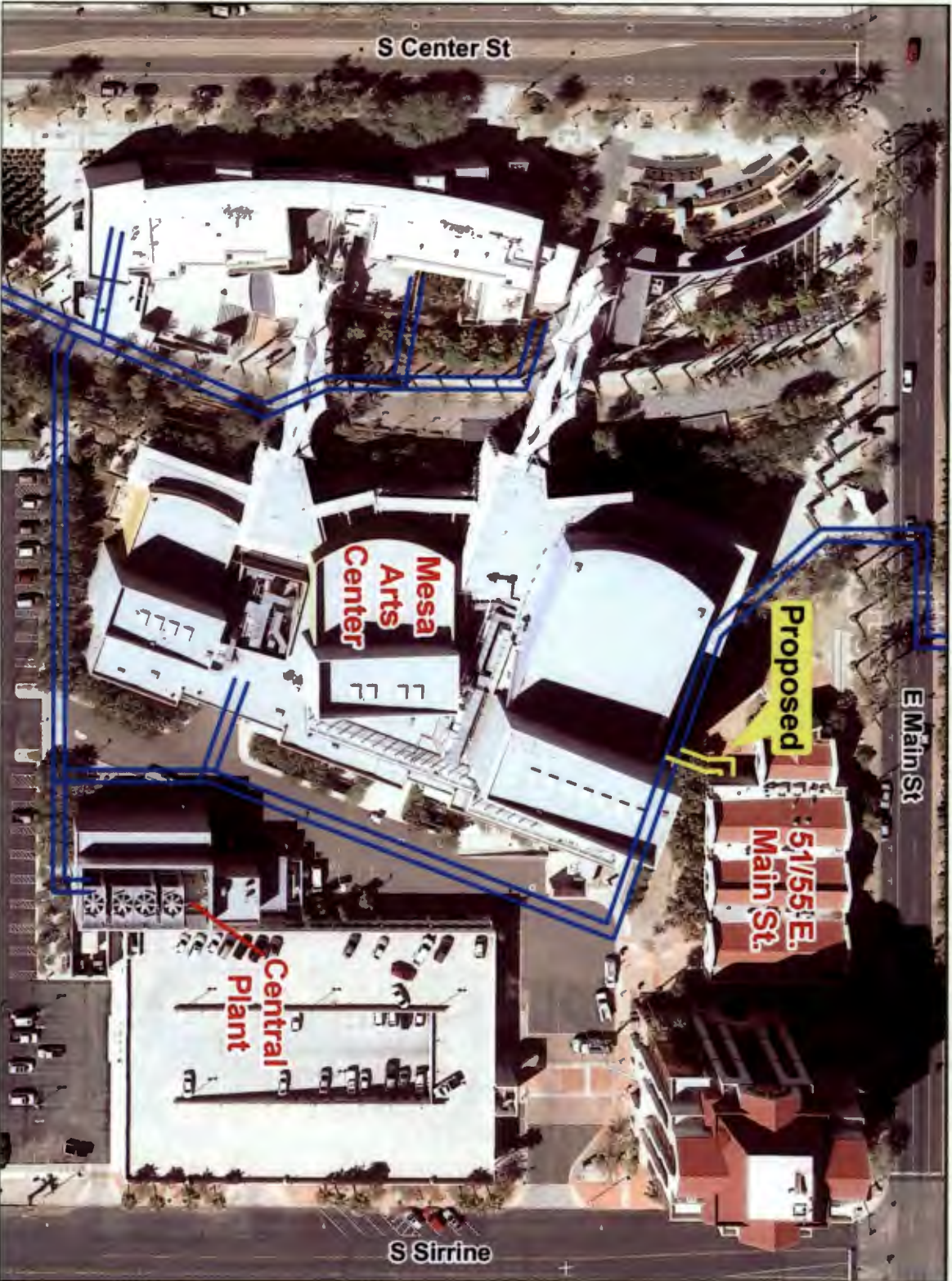
Mesa Arts Central Plant
