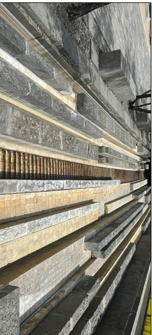
Mesa Arts Center Arroyo Refurbishing
