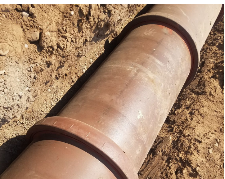
New Sewer Mains
