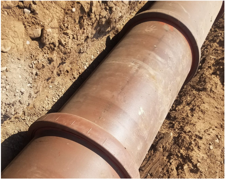
New Sewer Mains
