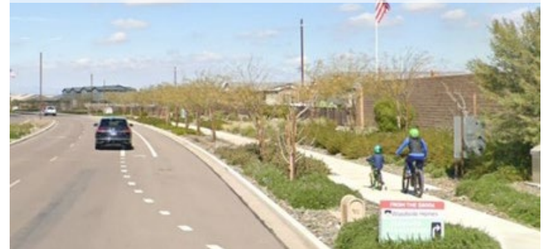
Bike lane is interrupted at intersection with no access available
